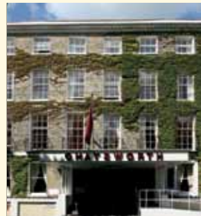
Chatsworth Hotel Worthing BN11 3DU
