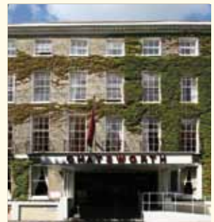
Chatsworth Hotel Worthing BN11 3DU
