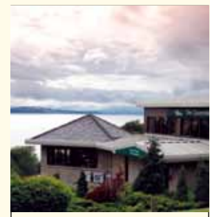
Queensferry Hotel North Queensferry KY11 1HP
